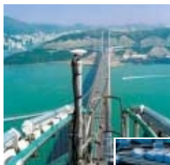
Bridge monitoring at Hong Kong with Leica CORS, GPS and GeoMoS
